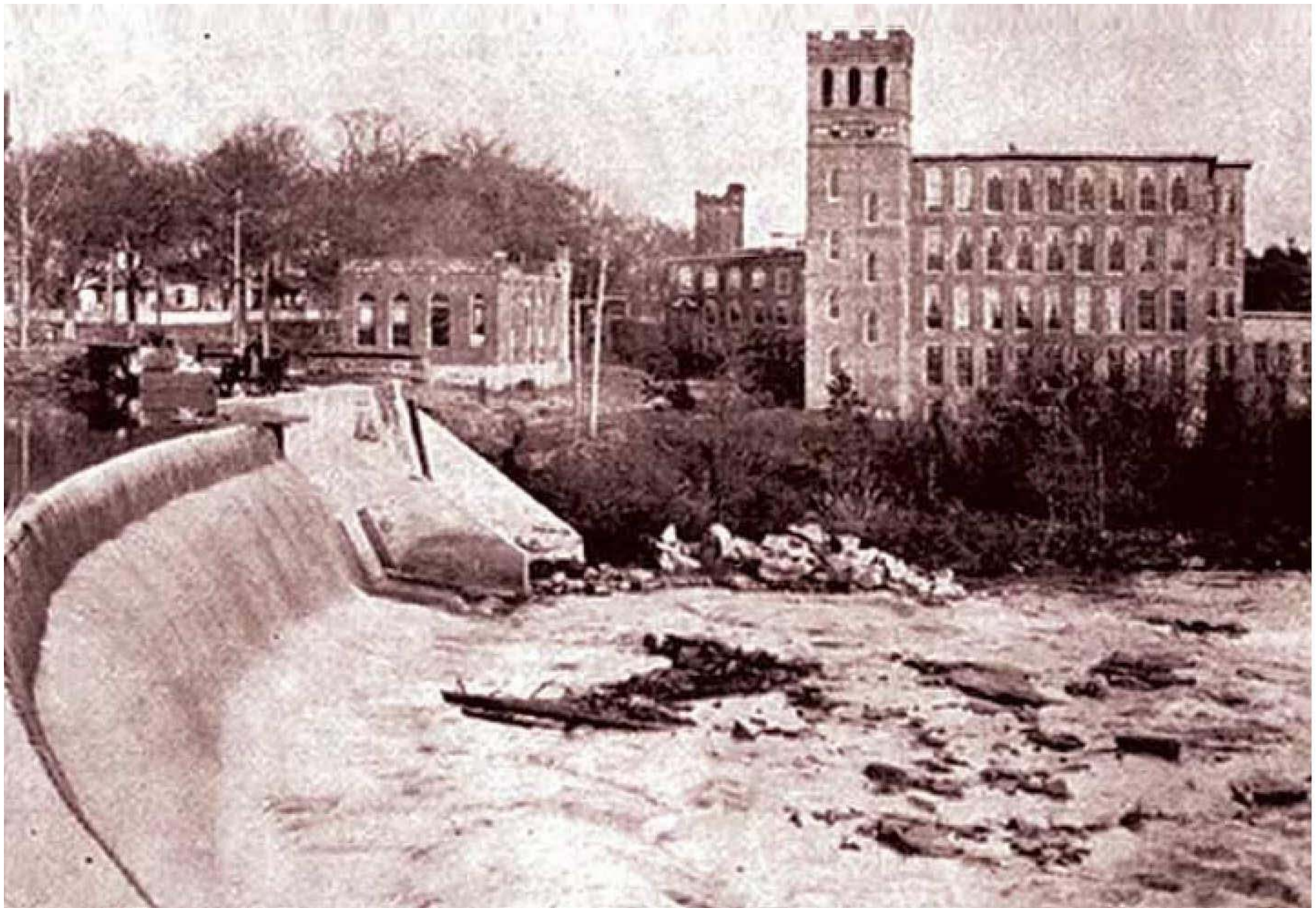
Glendale Mill around 1920
