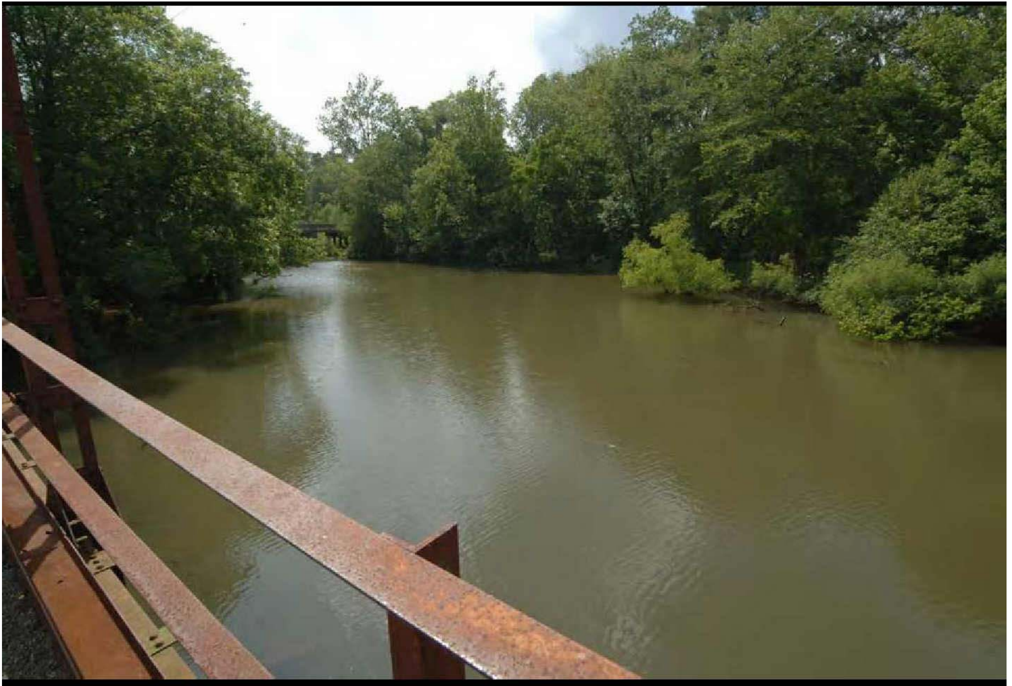
View of 1975 bridge from old iron bridge
