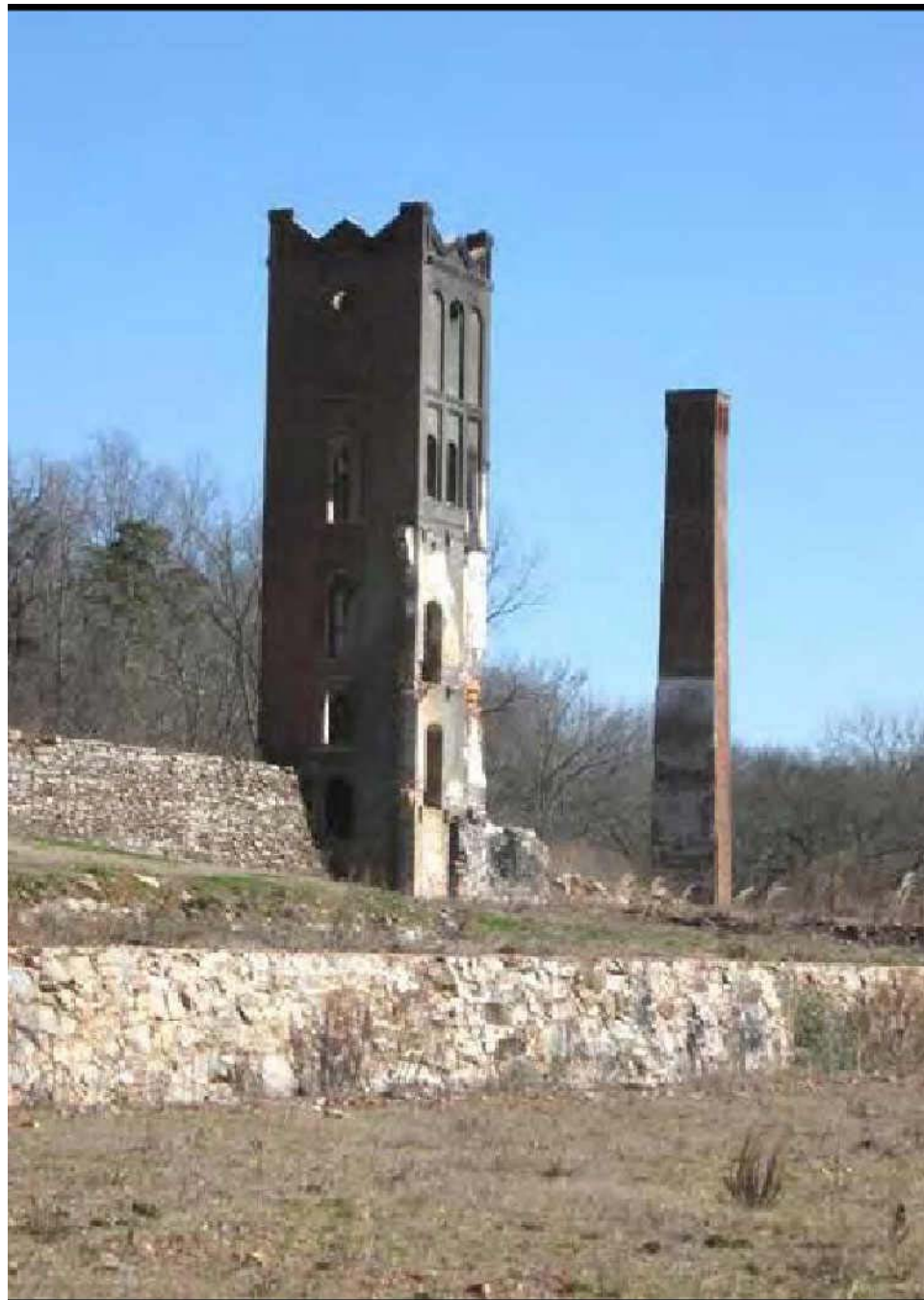
Small tower and older smokestack
