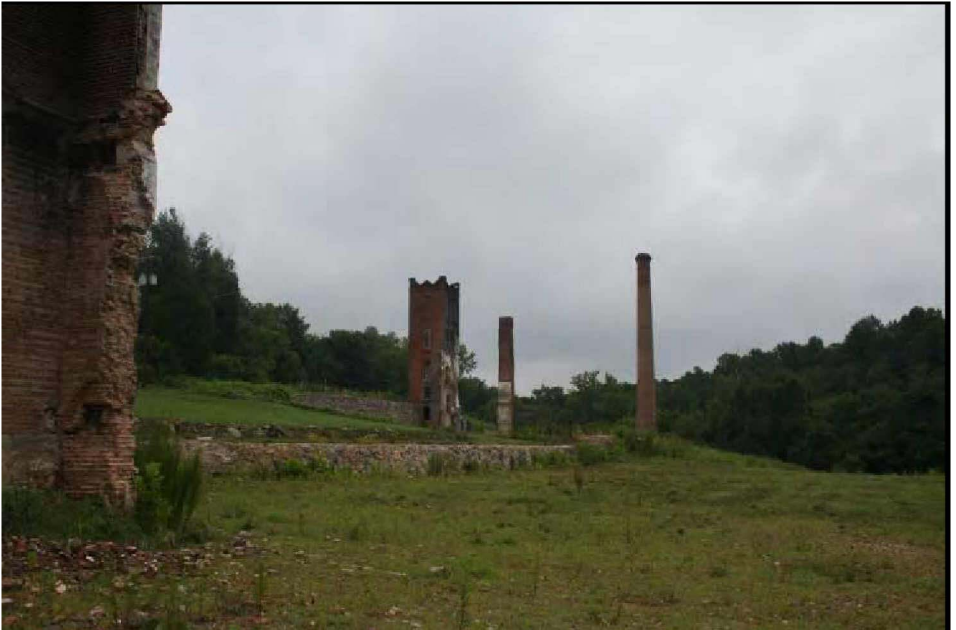
Mill site after fire and cleanup
