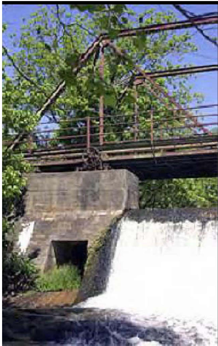
Bridge and dam
